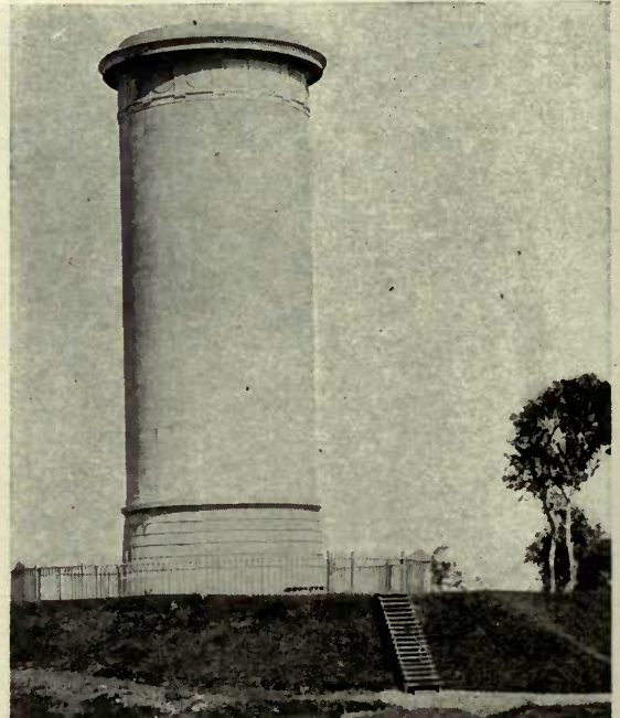
Concrete Stand Pipe Singson Water Works, Philippine Islands All concrete waterproofed with Truscon Waterproofing Paste, Concentrated.
